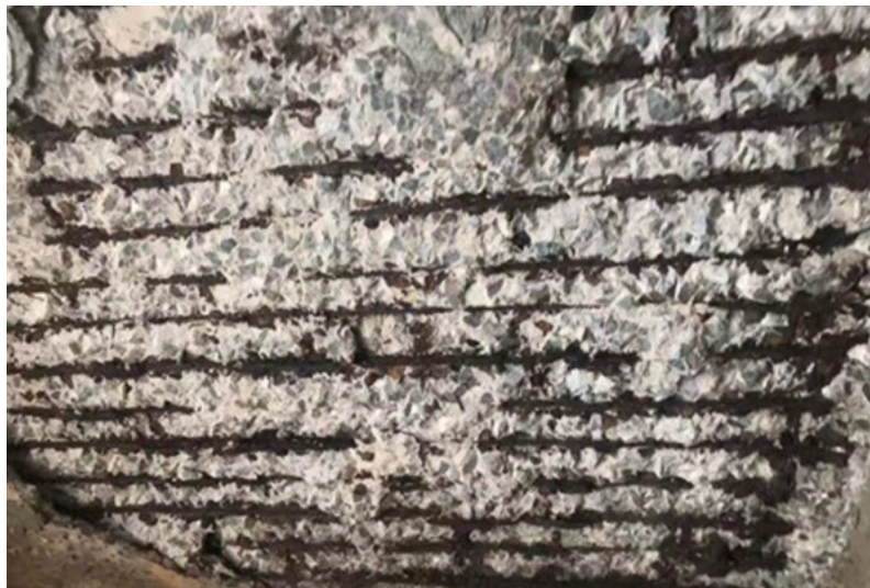
Rusting and peeling areas (front plate)
