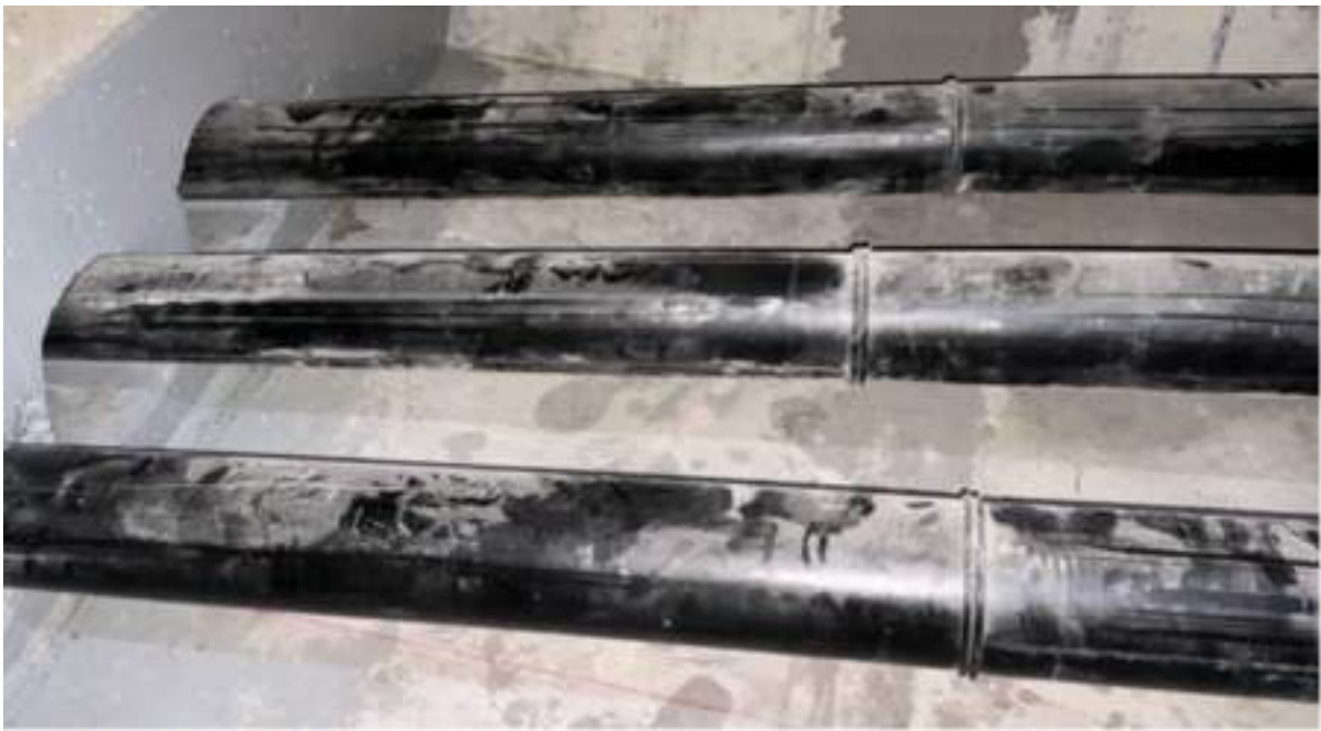
Figure 7: Anchorage and welding joints blockers
