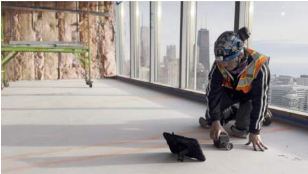
Photo courtesy of Zac Goodspeed / SafeCore Systems.
