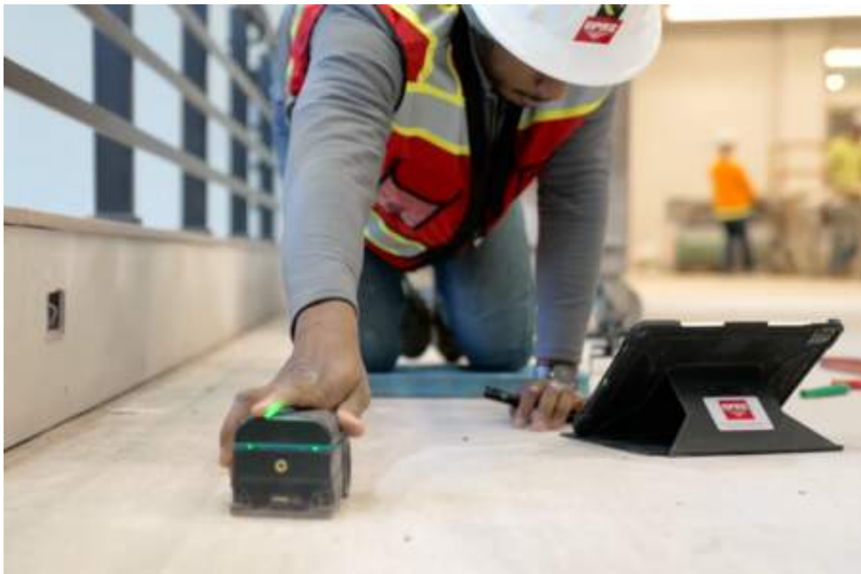
Photo courtesy of GPRS ( gp-radar.com )
