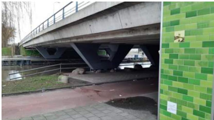
Side view of the bridge and drawings with indications of GPR data collection
