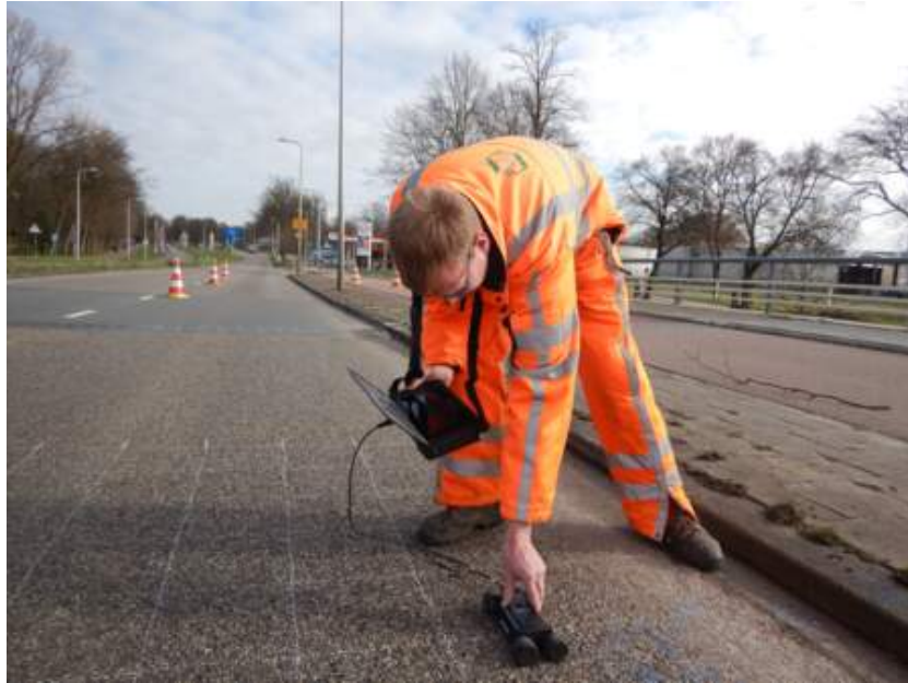
Using the Profometer on the bridge
