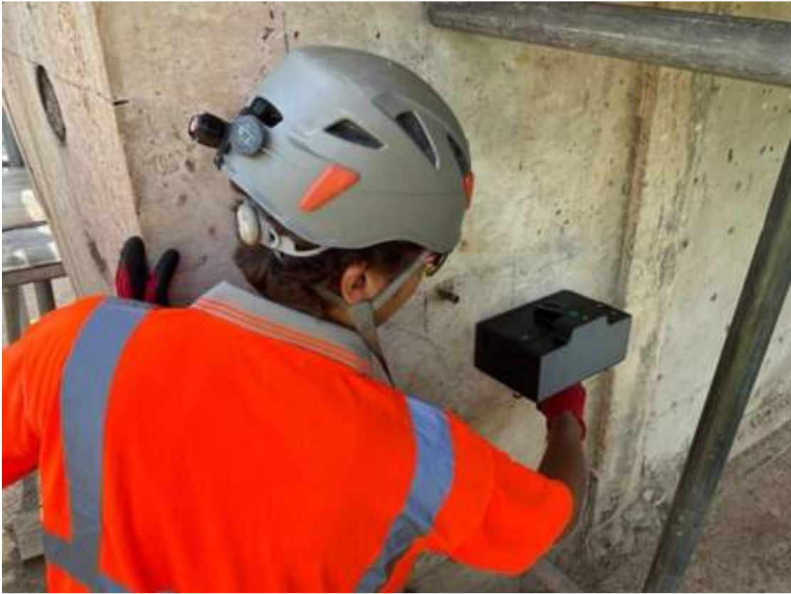
Non-destructive testing on the Huntingdon Railway Viaduct
