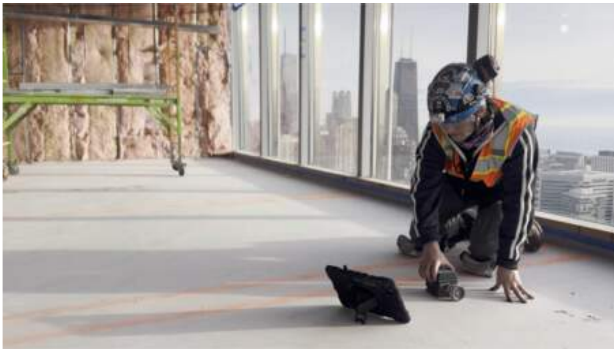
Photo courtesy of Zac Goodspeed / SafeCore Systems.
