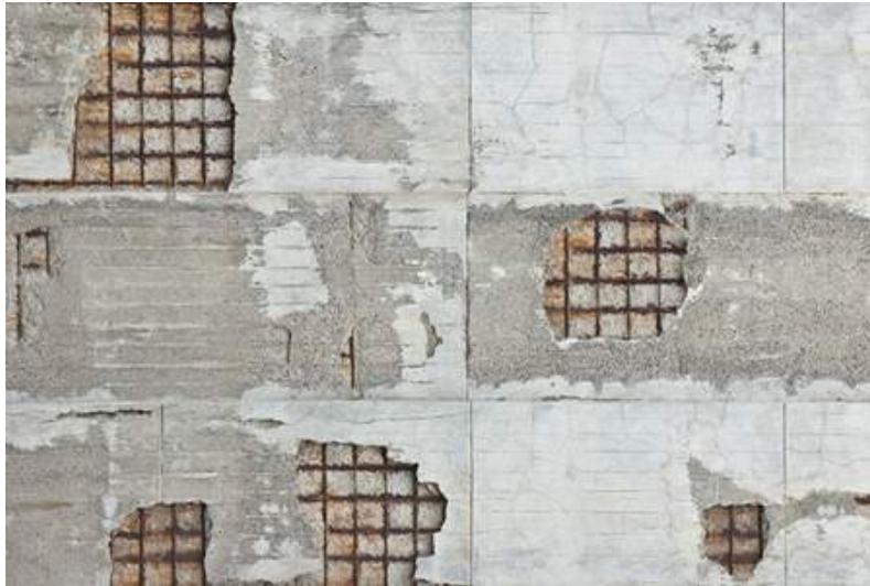
Concrete cover, homogeneity and concrete strength are the key parameters to determine if your structure is at risk of developing concrete cancer (corrosion, cracking, spalling, failure...).
