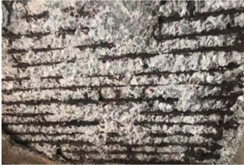
Rusting and peeling areas (front plate)
