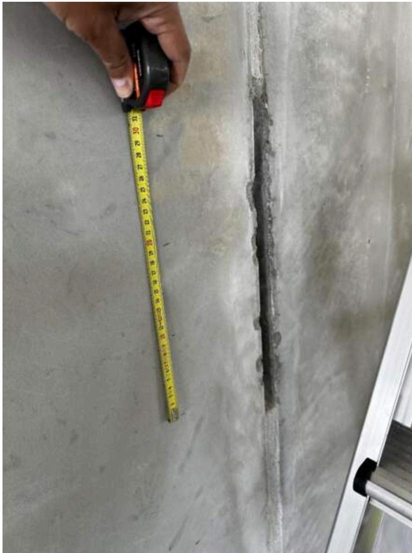
Voiding found over a 30cm length (they didn't break out the entire length of the void. Total length of voided joint section was estimated at 45cm)
