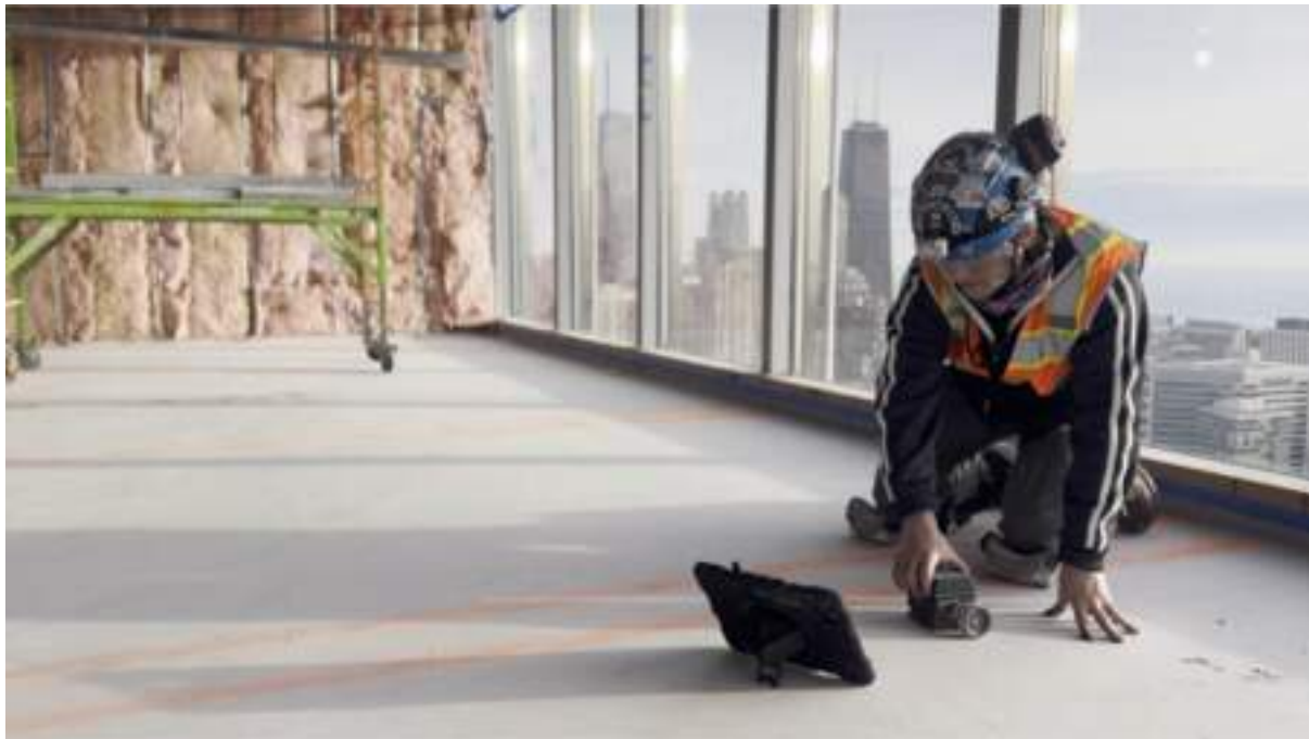
Photo courtesy of Zac Goodspeed / SafeCore Systems.
