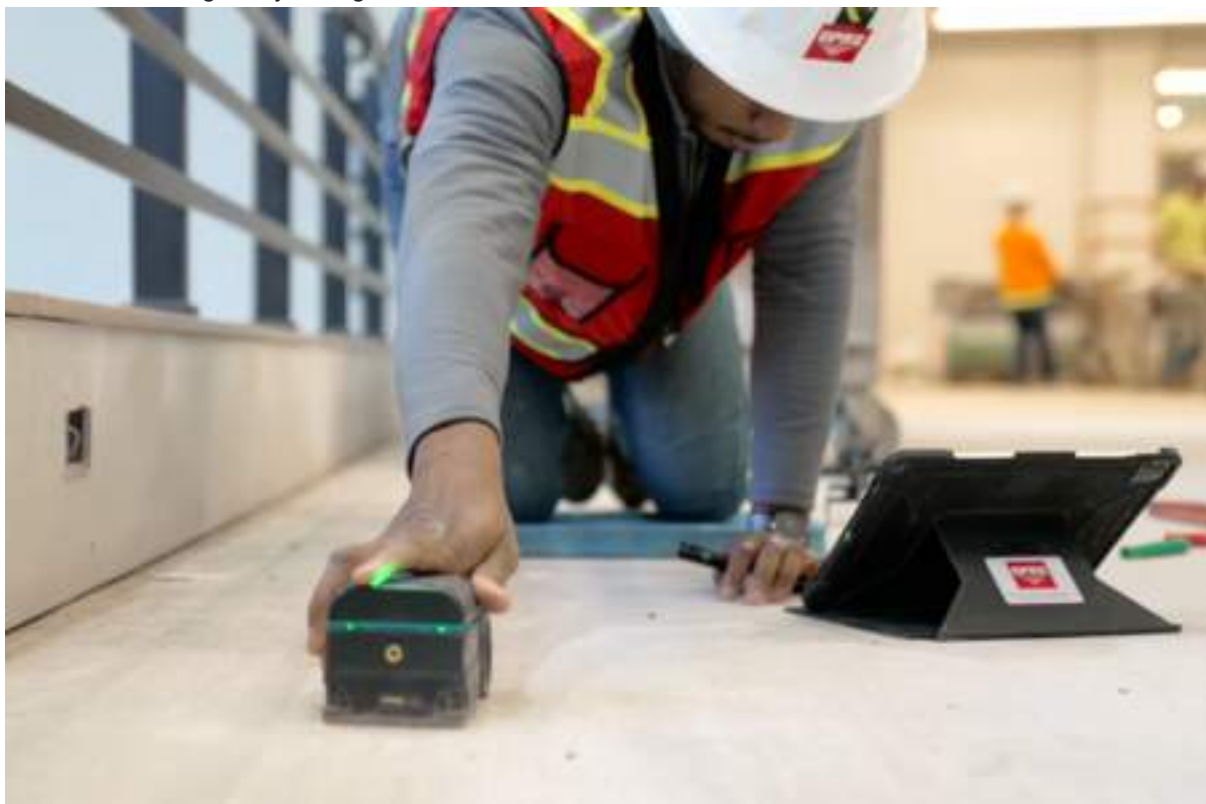
Photo courtesy of GPRS ( gp-radar.com )
