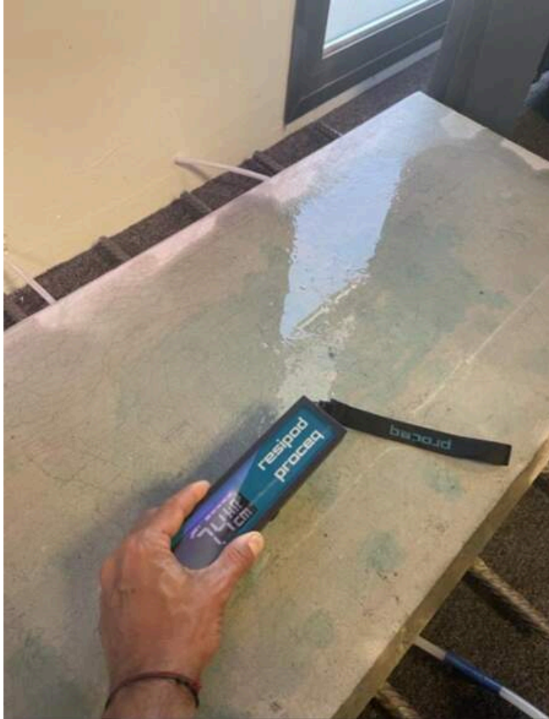
Concrete resistivity results using Resipod
