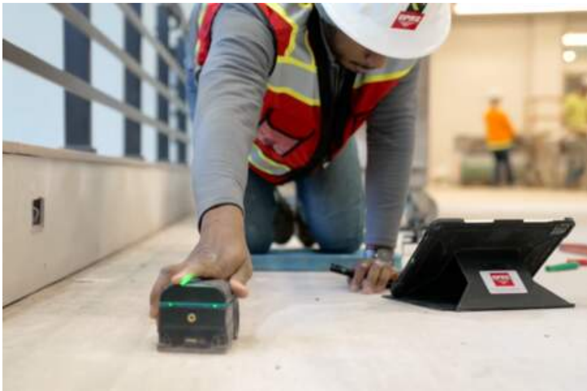
Photo courtesy of GPRS ( gp-radar.com )
