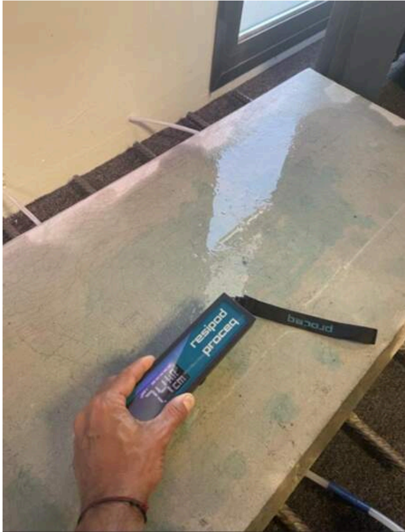
Concrete resistivity results using Resipod
