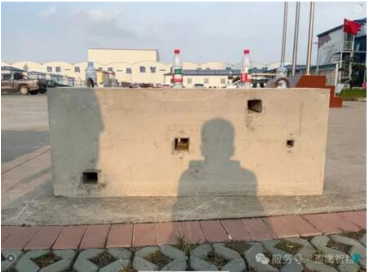
Back of test block
