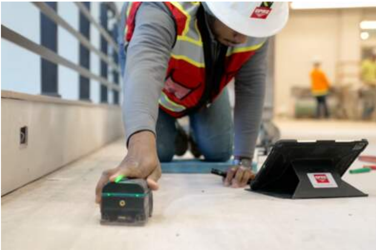
Photo courtesy of GPRS ( gp-radar.com )
