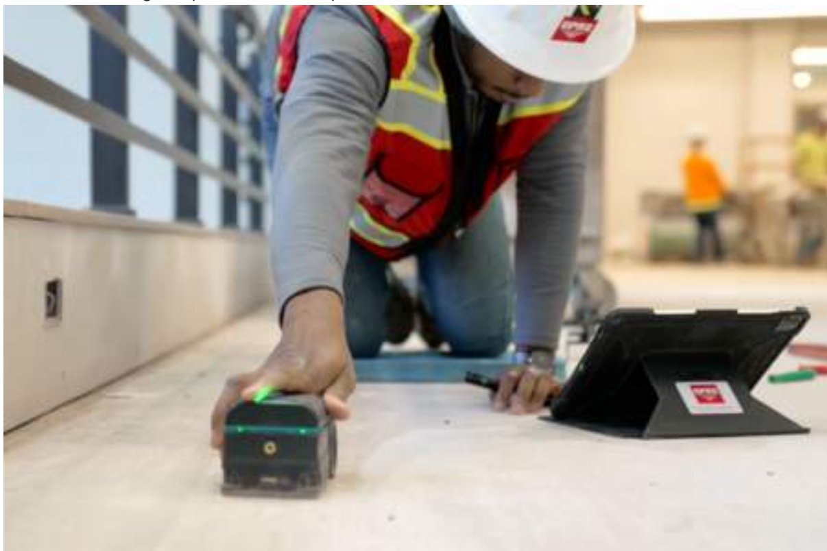
Photo courtesy of GPRS ( gp-radar.com )
