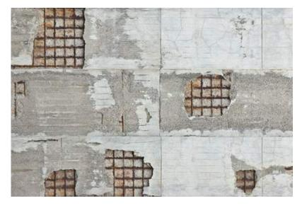
Concrete cover, homogeneity and concrete strength are the key parameters to determine if your structure is at risk of developing concrete cancer (corrosion, cracking, spalling, failure...).
