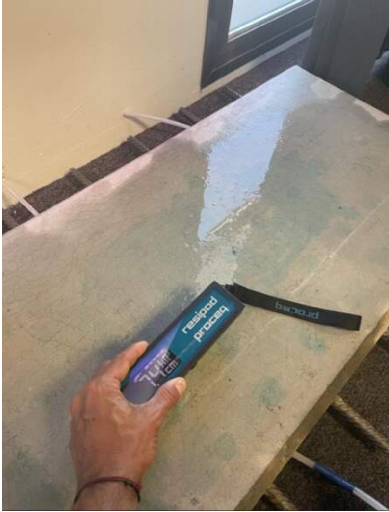
Concrete resistivity results using Resipod
