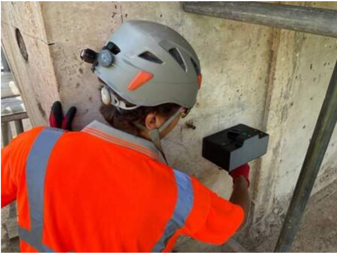
Non-destructive testing on the Huntingdon Railway Viaduct
